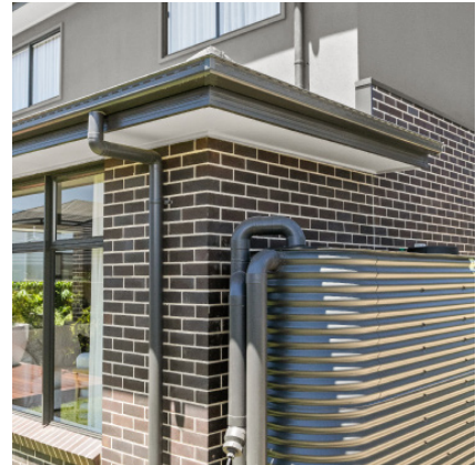
Above-ground rainwater tank
