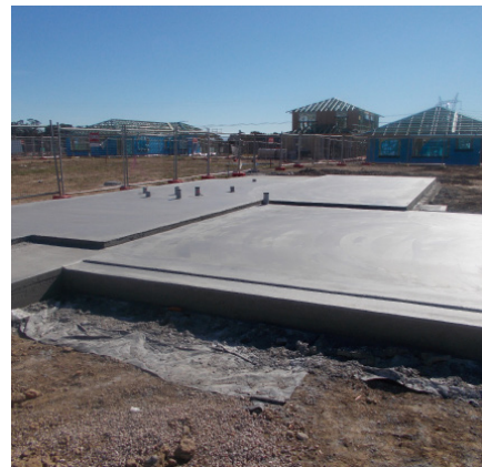
Waffle pod concrete slab
